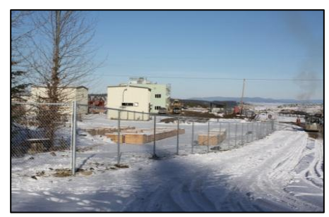
Mine Office/Warehouse Complete
