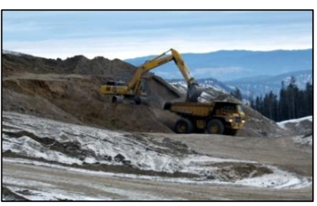
“Concentrator site preparation on schedule”
