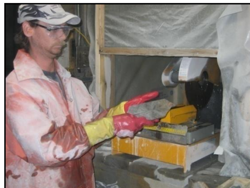
Core cutting is done on site
