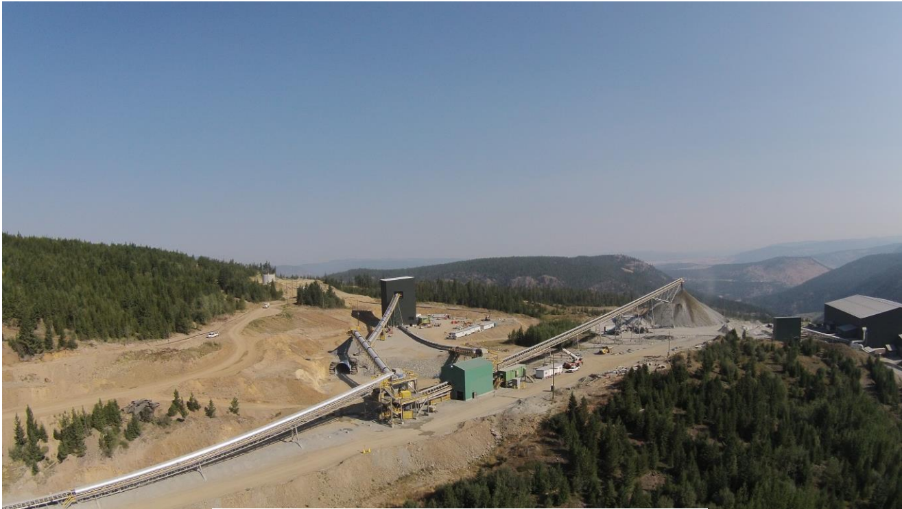
Aerial View of Completed Secondary Crusher Installation
