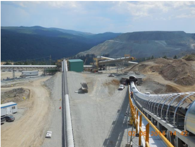
View from Secondary Crusher Building
