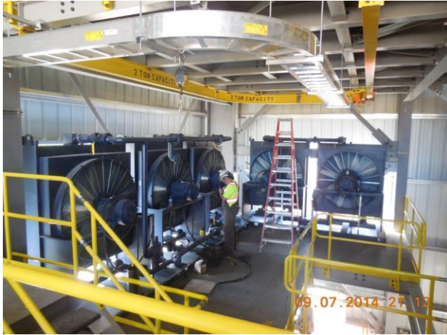
Installation of cooling fans
