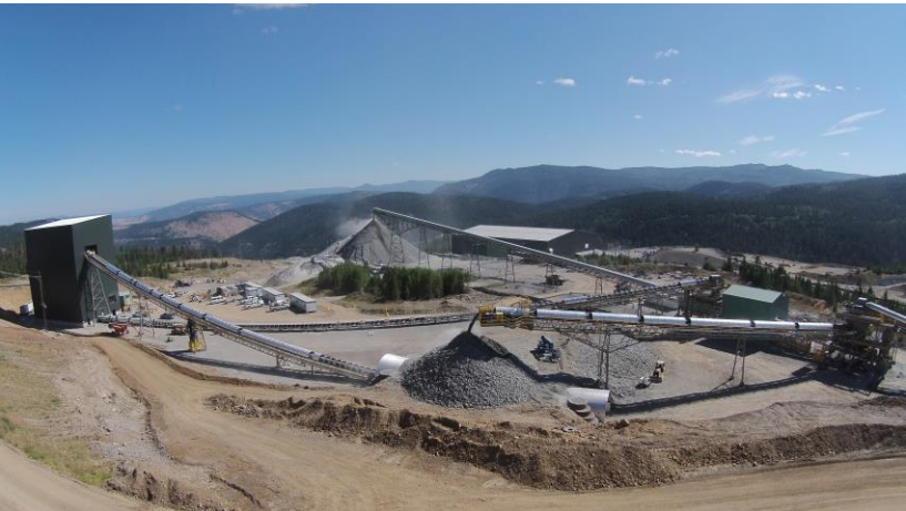
Secondary crusher in operation - Aug 6-2014
