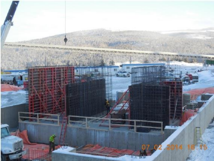
Rebar installation for lower bowl foundation base
