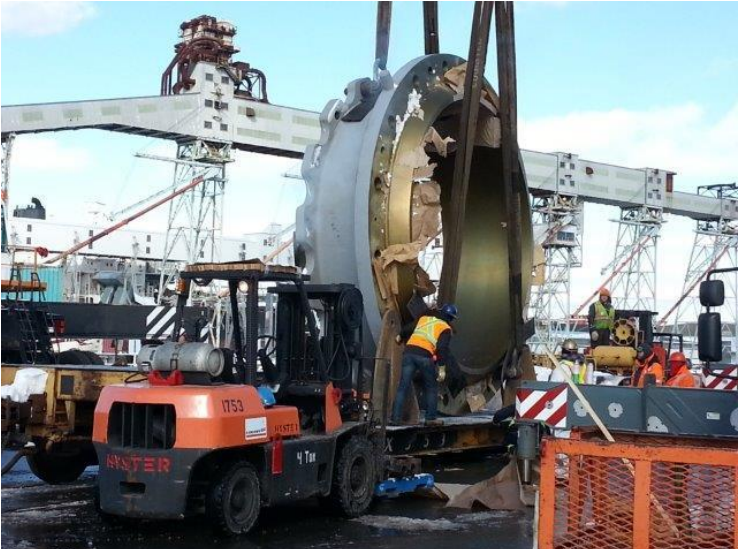
Unloading of adjustment clamping ring assembly at the port of Halifax
