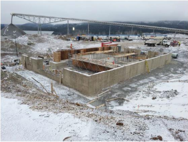
Foundation work for secondary crusher at mine site
