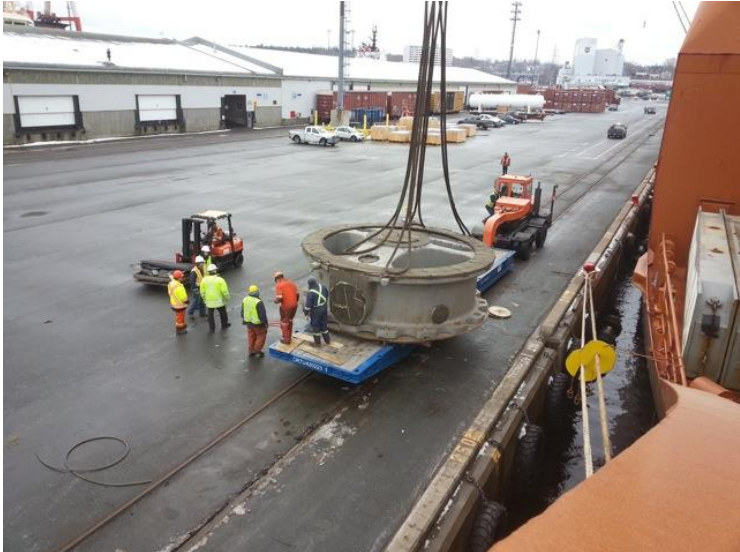
Unloading of lower main frame assembly at the port of Halifax
